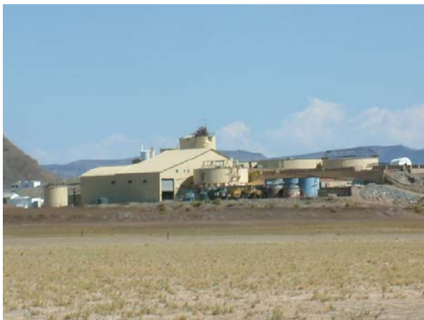
Columbus Mill Site Building – July 1 st , 2008
