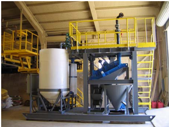
Installation of Module 1 of our Pilot Plant
