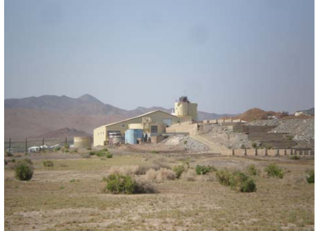
Columbus Mill Site Building – July 1 st , 2008
