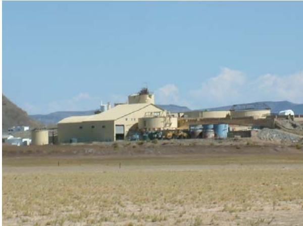
Columbus Mill Facility – July 1 st , 2008
